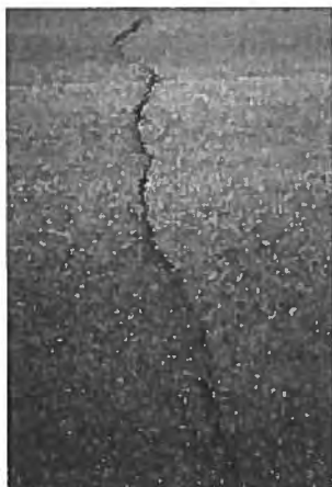
▲ Tight cracks less than \frac{1}{4} " in width.
