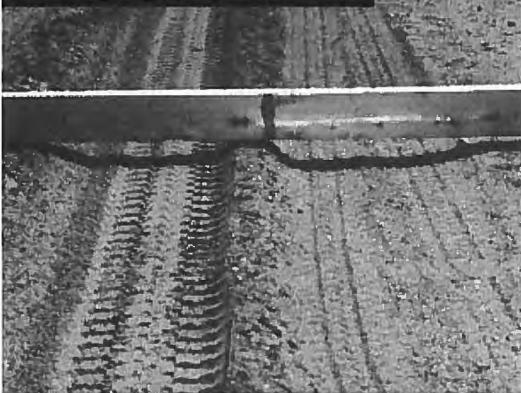
Moderate ruts in soft dry soil surface. Periodic maintenance grading helps improve ride and access.
