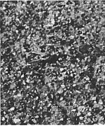
Severe raveling with ▼ extreme loss of aggregate.
