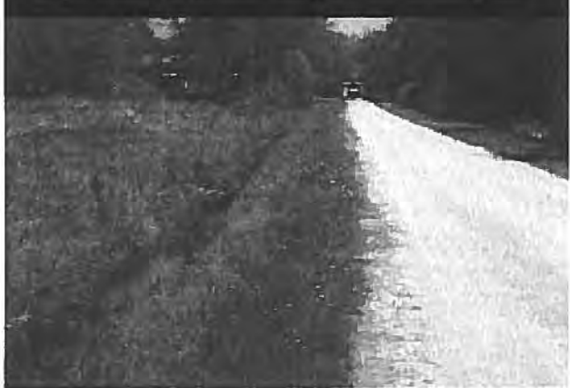
A ditch has been constructed along this soil-surfaced road.
