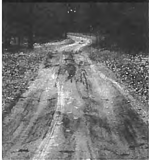
Moderate rutting in low area where water crosses an ungraded road.
