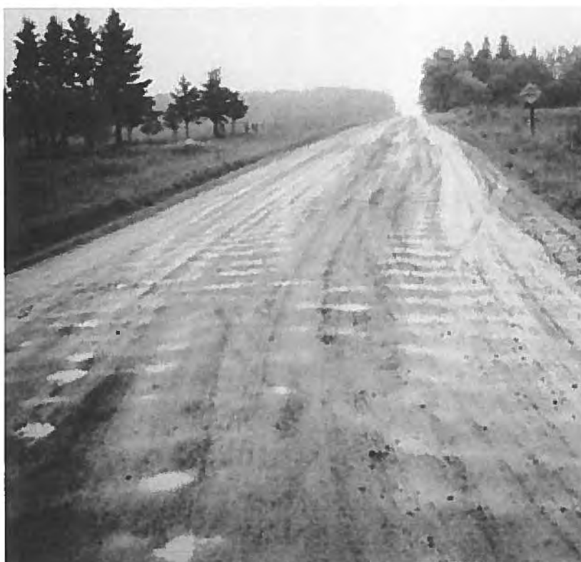
► Severe washboarding traps water.
