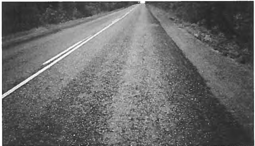
► Moderate to severe raveling in wheel paths.
