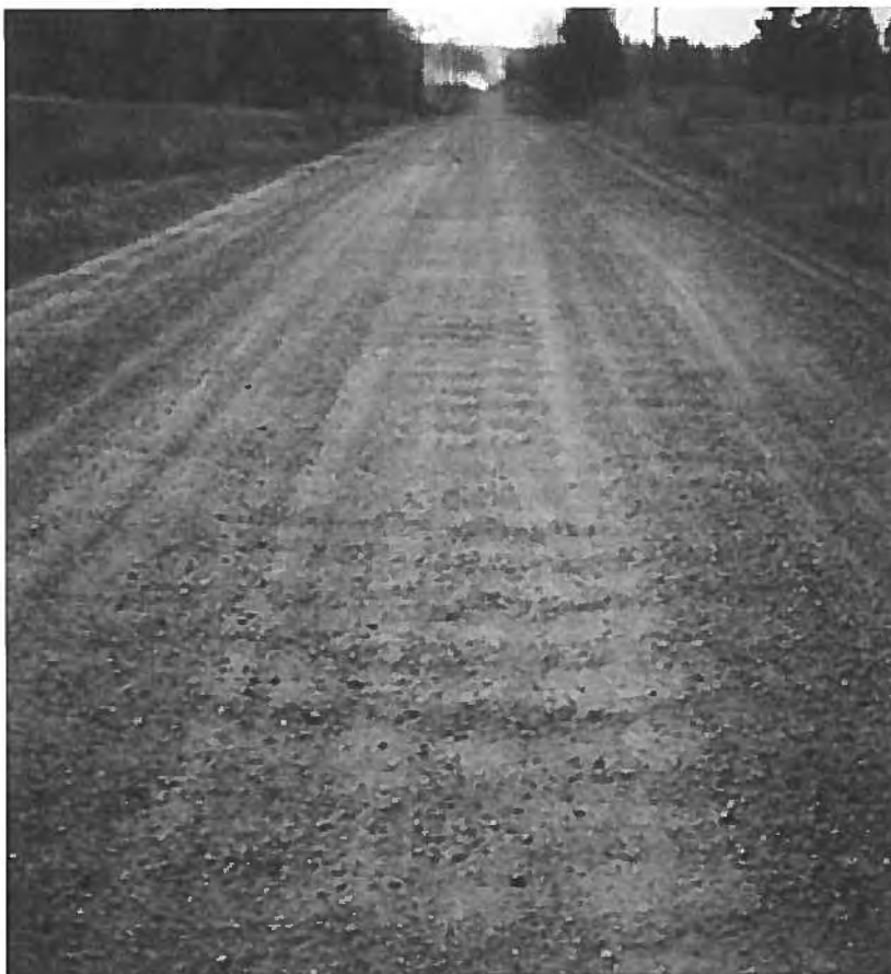
▼ Moderate washboarding in center of road.
