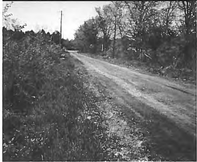
Narrow road to a single property has a graded crown and ditch for drainage.
