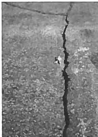
▲ Open crack – \frac{1}{2} " or more in width.
