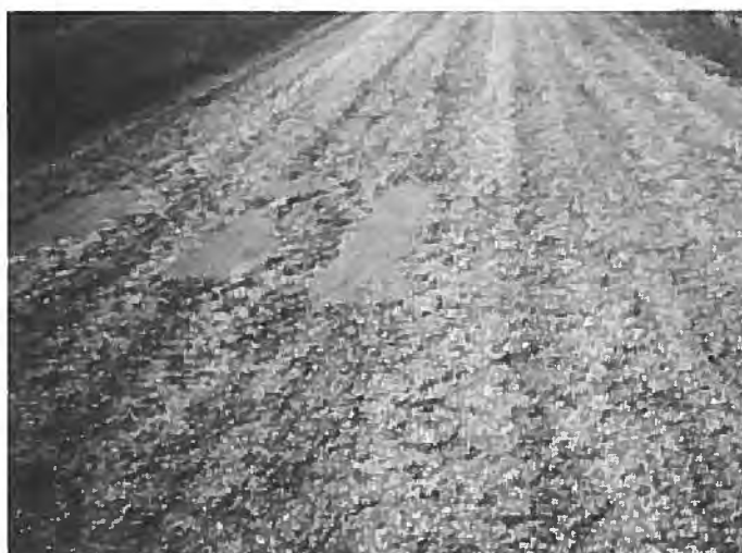
◀ Severe raveling and loss of surface material.
