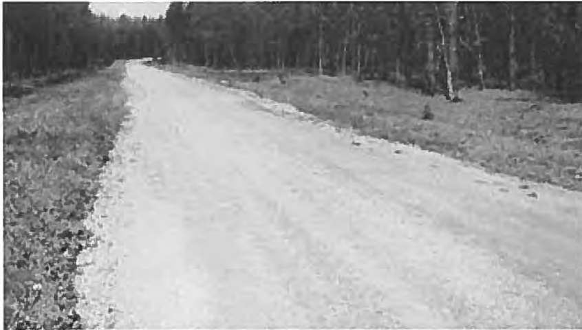
◄ Adequate gravel layer. No ruts or potholes.
