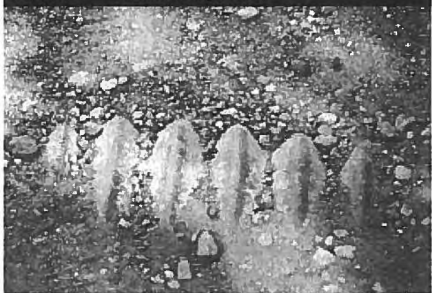
Shallow culvert is provided. Prevents water from crossing the road. More fill is desirable to protect culvert from traffic.
