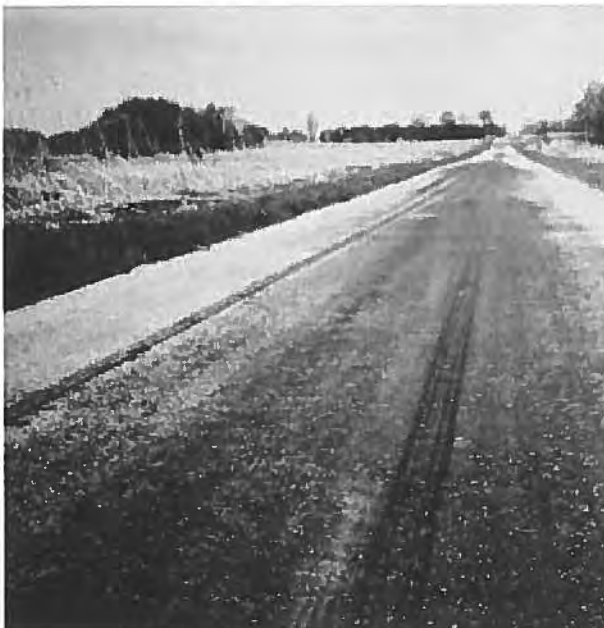
▼ Severe flushing.
