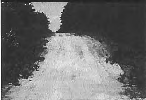
Road follows natural terrain. No grading with cuts or fills. Comfortable ride less than 10 mph.
