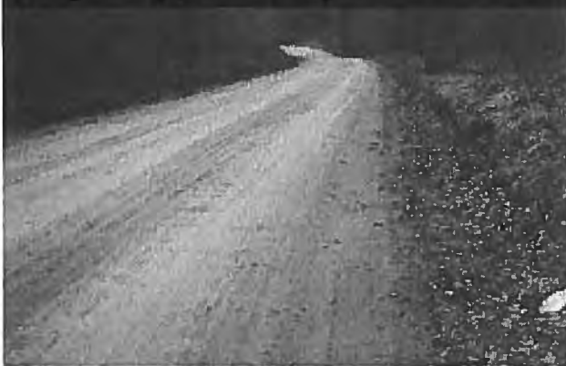
This graded road with sandy soil has a crown for improved drainage. Driving speeds over 30 mph are comfortable.
