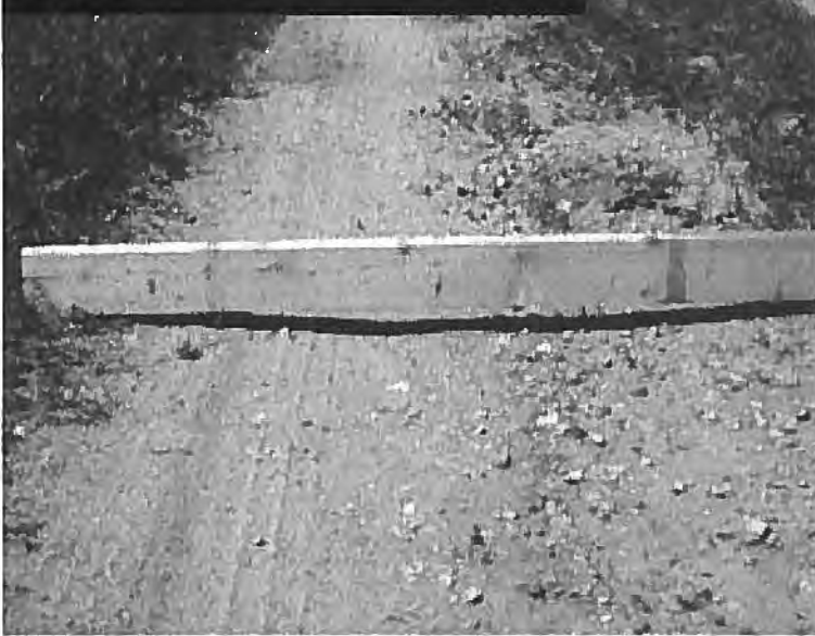
Slight ruts in wheel path.
