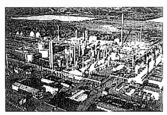
Natural gas is extracted through a drilling process. The photo on the right shows a typical drill size for natural gas extraction. Natural gas also has to be processed. The processing consists of separating all of the various hydrocarbons and fluids from the pure natural gas, to produce what is known as 'pipeline quality' dry natural gas. The photo on the right shows a typical natural gas processing plant. This is allowed as a conditional use within the M-R zone.
